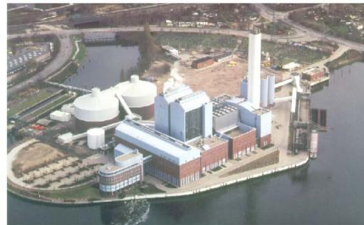
Fig. 1. The Tiefstack Power Plant in Hamburg featuring two 50,000 m<sup>3</sup> Eurosilos
